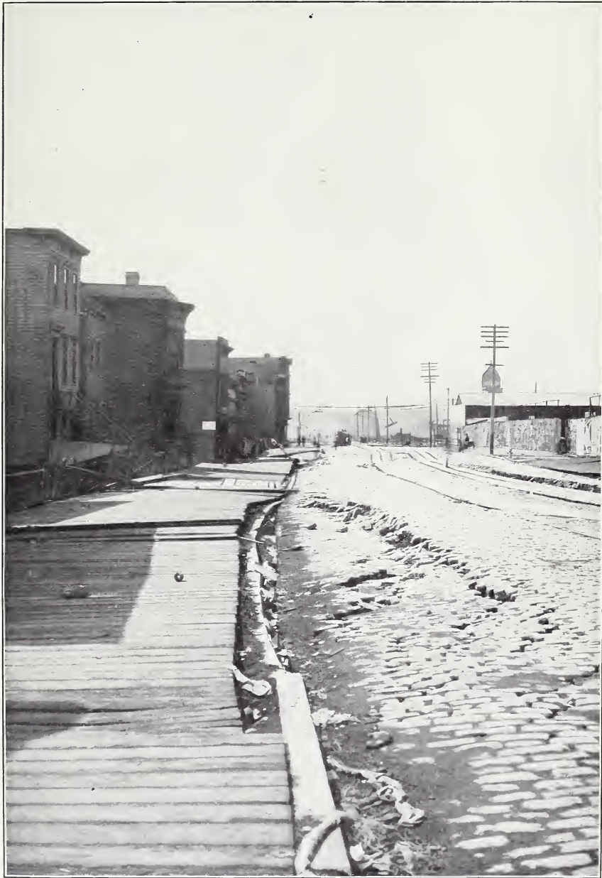
RESULTS OF EARTH FLOW, NINTH STREET, SAN FRANCISCO.
